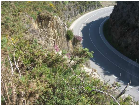
Figure 4: Photo of the studied road
